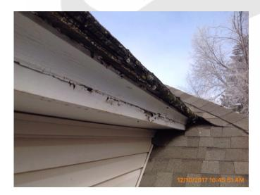
There are presently multiple layers of roofing materials applied over this structure. When the roof is replaced, at least the top layer will have to be removed. Requirements vary between jurisdictions as to the maximum number of layers permitted.
